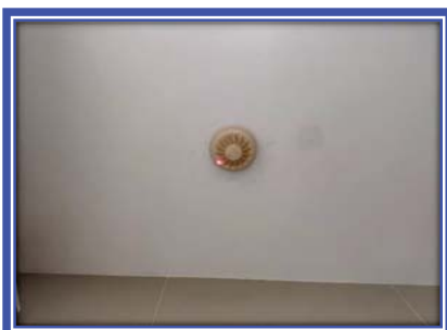
Picture shown : Testing the heat detector and then the device is working properly.
