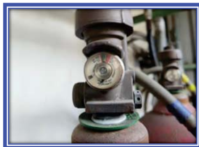
Figure 4 Picture show the pressure gauge for Inergen cylinder number 4
