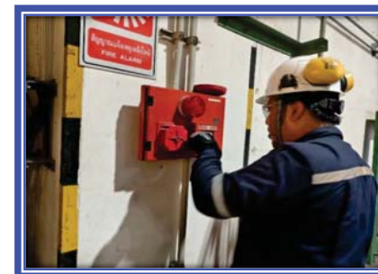
Picture shown : Function test crosszone the preaction system working properly.
