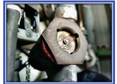
Picture shown : The solenoid valve of inergen system working properly.
