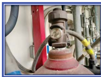
Figure 16 Picture show the pressure gauge for Inergen cylinder number 16
