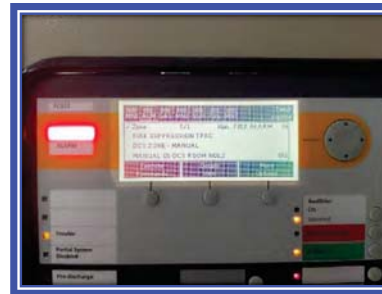
Picture shown : Function test cross zone detector and control panel and graphic annunciator working properly.
