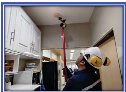
Picture shown : Testing the heat detector and then the device is working properly.
