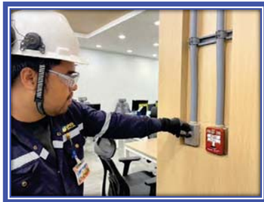
Picture shown : Function test abort switch and all device working properly.
