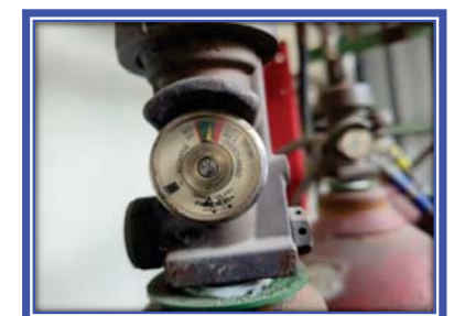
Figure 12 Picture show the pressure gauge for Inergen cylinder number 12
