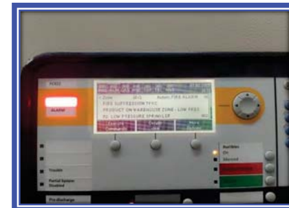
Picture shown : Function test low pressure switch and control panel working properly.
