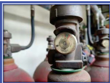
Figure 5 Picture show the pressure gauge for Inergen cylinder number 5
