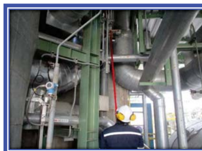
Picture shown : Testing the heat detector and then the device is working properly.
