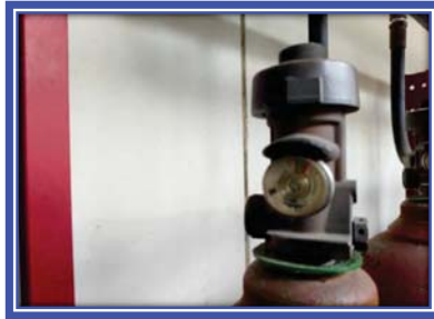
Figure 2 Picture show the pressure gauge for Inergen cylinder number 2
