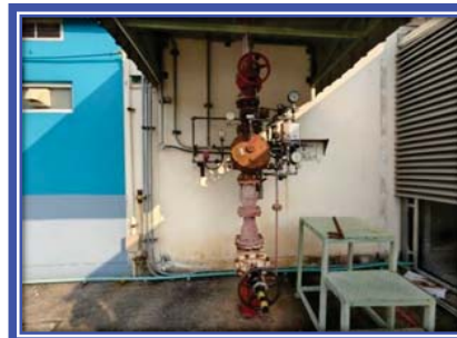
Picture shown :Inspection preaction system before function test at product warehouse building.
