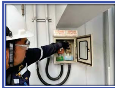
Picture shown : Function test abort switch and all device working properly.
