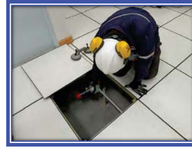
Picture shown : Testing the smoke detector of inergen system.
