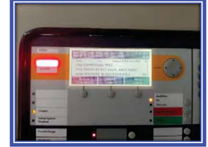
Picture shown : Function test pressure switch and control panel working properly.
