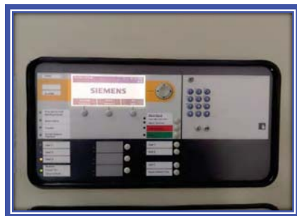
Picture shown : Return the preaction system in normal condition.
