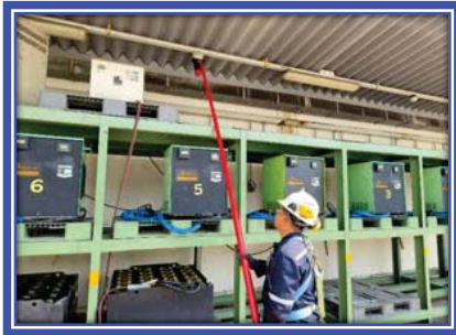
Picture shown : Testing the fire alarm system and the control panel is working properly.
