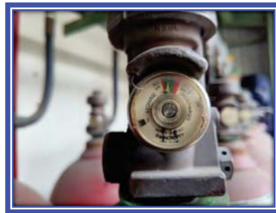
Figure 14 Picture show the pressure gauge for Inergen cylinder number 14
