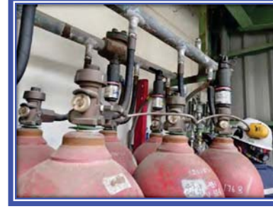
Picture shown : Cleaning and return inergen system to normal condition.
