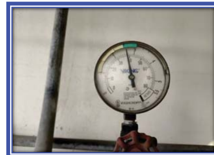
Picture shown :Inspection preaction system before function test at product warehouse building.
