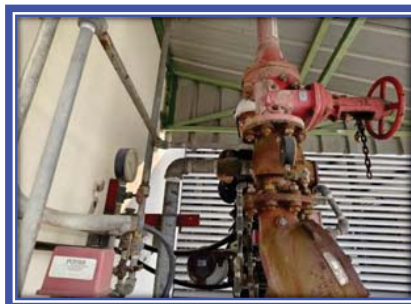
Picture shown : Function test crosszone the preaction system working properly.
