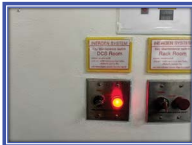
Picture shown : Function test key maintenance switch and key bypass switch all device working properly.
