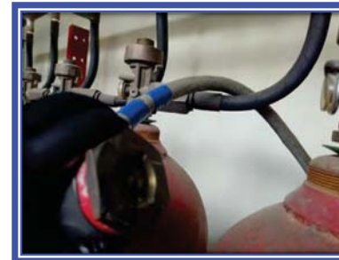
Picture shown : The solenoid valve of inergen system working properly.
