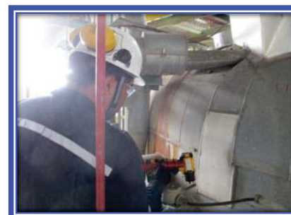
Picture shown : Testing the heat detector and then the device is working properly.
