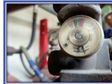
Figure 9 Picture show the pressure gauge for Inergen cylinder number 9
