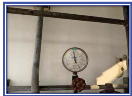
Picture shown : Return the preaction system in normal condition.
