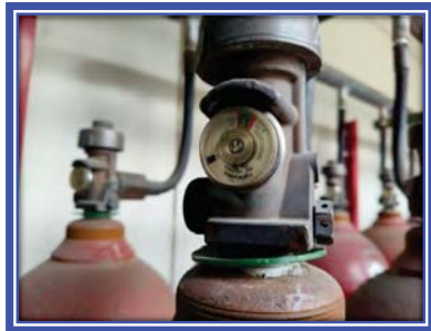
Figure 13 Picture show the pressure gauge for Inergen cylinder number 13
