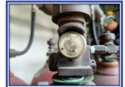
Figure 10 Picture show the pressure gauge for Inergen cylinder number 10
