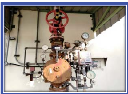
Picture shown : Return the preaction system in normal condition.
